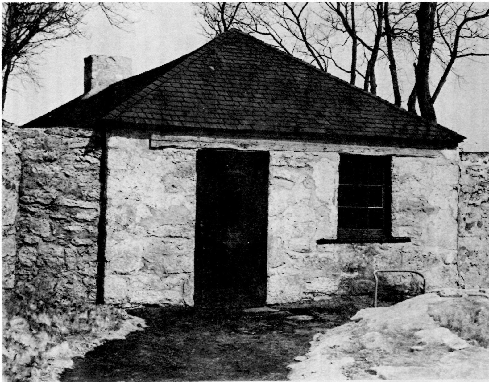
AS FOUND BAKE HOUSE LOWER FORT GARRY, SELKIRK, MANITOBA
